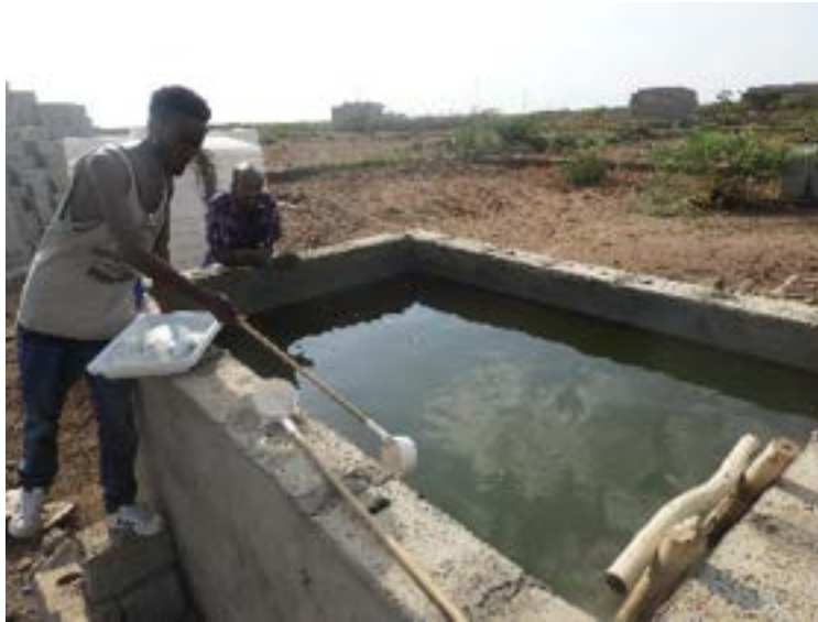
Figure 2b. Concrete cistern in Ethiopia
